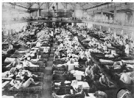
Heliopolis Hospital, Egypt c1915
